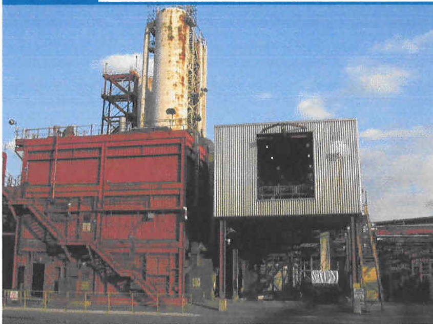
Filter press building.
